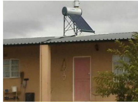
Figure 18: Solar geysers at Ysterfontein worker's houses
